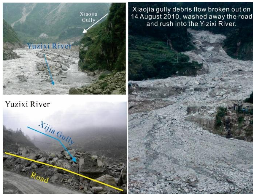
Figure 2 The Xiaojia Gully Debris Flow Outbreak in August 14, 2010 Flooded the Blocking Dam and the Highway
